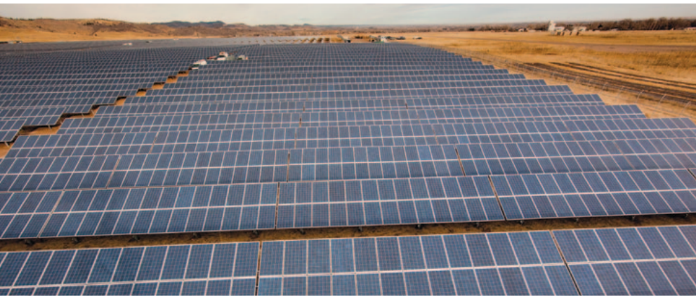
Left: This 3,300 kilowatt array, located on Colorado State University’s Foothills Campus, generates five million kilowatt hours annually and spans 30 acres. Photo courtesy of Dan Bihn. Right: The Student Recreation Center at Colorado State University has undergone a complete renovation. The cost of energy within the renovated building is less than before despite an addition of 75,000 square feet. Photo courtesy of Becca Wren
